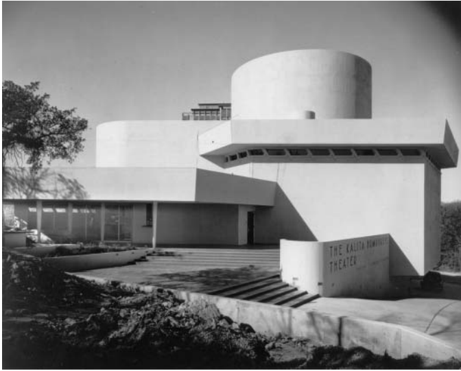
17 Wright, Kalita Humphreys Theater, view from southeast, after imperfections and formwork marks were removed and the surface was painted, late 1959 or early 1960. FLWA, photograph no. 5514.0023 (artwork all rights reserved The Frank Lloyd Wright Foundation Archives [The Museum of Modern Art | Avery Architectural & Fine Arts Library, Columbia University, New York]; photograph by Messina Studios)
